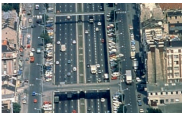
Photo 3 - Autoroute A1 avant requalification.
